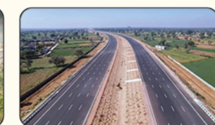
NEAR 8 LANE EXPRESS HIGHWAY
