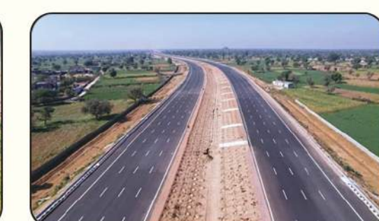
NEAR 8 LANE EXPRESS HIGHWAY
