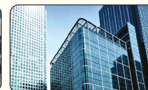
BEHIND L&T DATA CENTER
